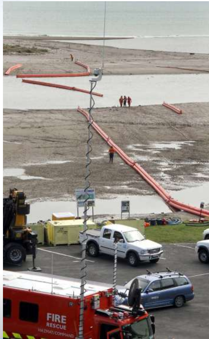
Booms being deployed at Maketu Estuary – 22 October
